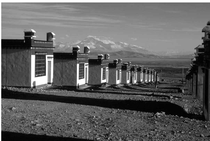
A new settlement site for Tibetan nomads in Darchen, in Ngari Prefecture (Chinese: Ali) in the Tibet Autonomous Region (TAR). Often new settlements, like this one, are far from community resources.
